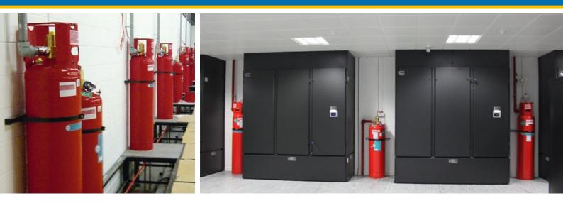
The design standards for fire suppression systems within a server room and data centre have been developed with strict guidelines to help ensure the safety of the system. Design considerations such as the position of cylinders, piping and nozzles, to ensure quick response times, also play a key role when selecting the most effective fire suppression solution for this type of environment.
